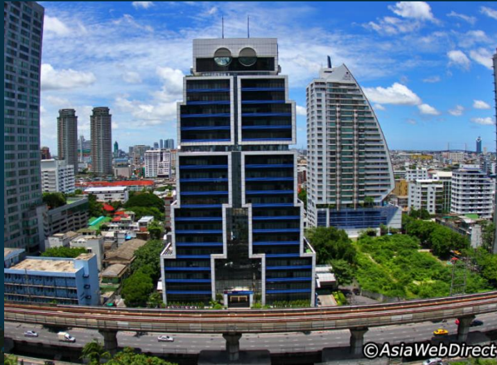
UOB ROBOT BUILDING
